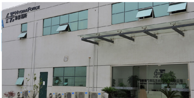
ASIAN/PACIFIC HEADQUARTERS, PRECISION MACHINING AND MANIFOLD ASSEMBLY FACILITY IN CHANGZHOU, CHINA, NEAR SHANGHAI.
