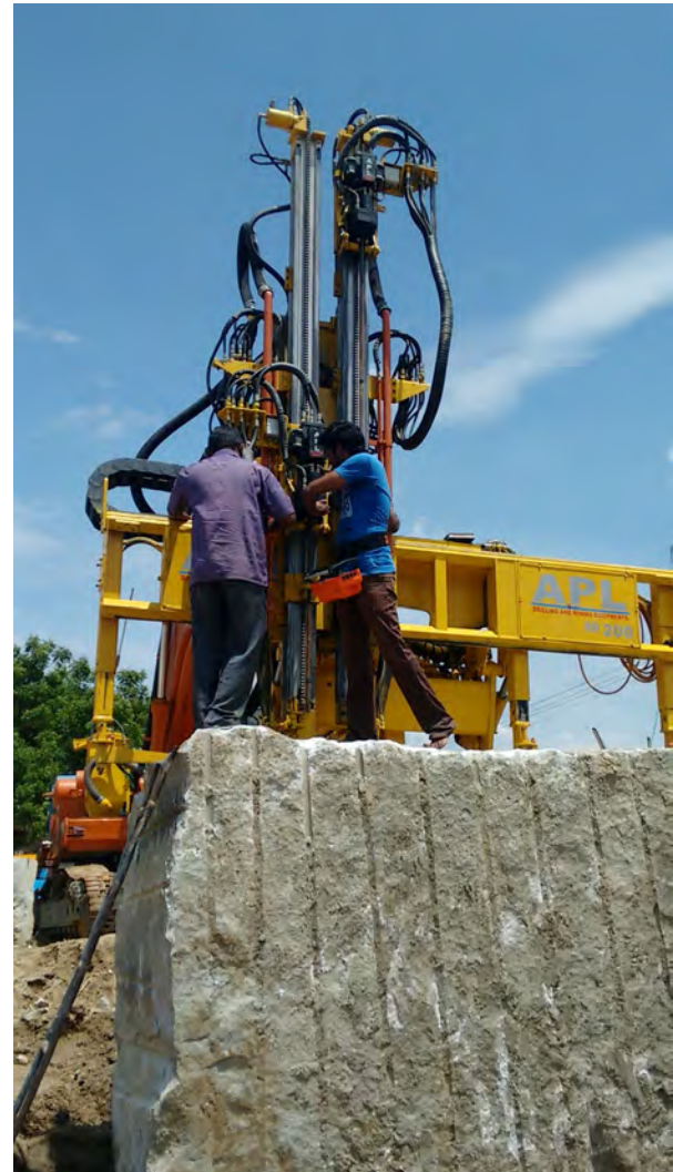
Setting the system for Drilling using Radio Remote
